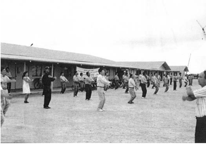
Figure 9.5 Gymnastic exercises at the site
