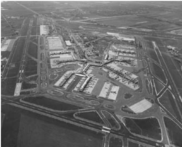
Figure 7.1 Aerial view of Schiphol Airport
