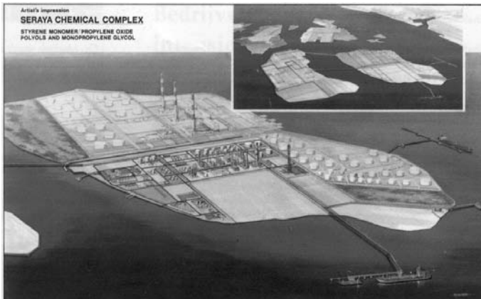
Figure 9.3 An aerial view of Seraya Chemical complex (Shell Venster, 1994, p.21)
